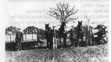
Hunsbury Hill Quarries. A posed photograph of a Wagon team at Green Lane crossing, 19011, showing loaded and empty wagons, horses, drivers and brakesmen.
